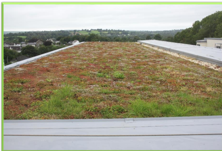
Living roofs can be used to mitigate habitat loss, stabilise heating and sound within a building and contribute to decarbonisation
