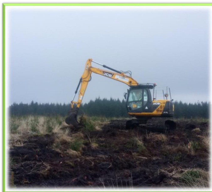
Ground smoothing techniques to restore functioning peatland
